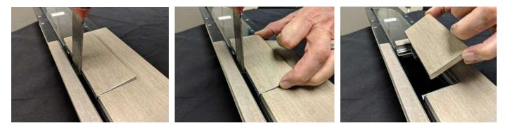
1. Remove the Access Cover by pushing down on the black tab at the center of the Access Cover with a screwdriver, putty knife, or similar tool. The Access Cover will pop up and allow you to grab and remove it.
