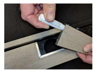
7. Before re-installing the Access Cover apply wax or petroleum jelly around perimeter to aid in future removal.
