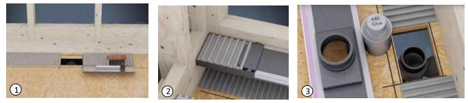
Use a spirit level to verify that the INNI is absolutely level. Adjust the INNI as needed to ensure a level installation. If the INNI is not leveled, it won't drain properly.
