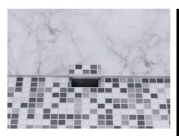
Re-Install the Access Cover Tray by angling the cover down to the Drain Channel until the ball detents catch the Access Cover Frame. Push the cover down until flush.
