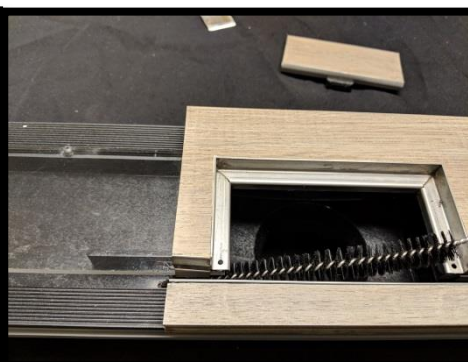
4. Use the cylindrical brush to clean along the inlet slot.
