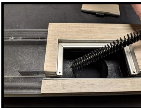
4. Use the cylindrical brush to clean along the inlet slot.
